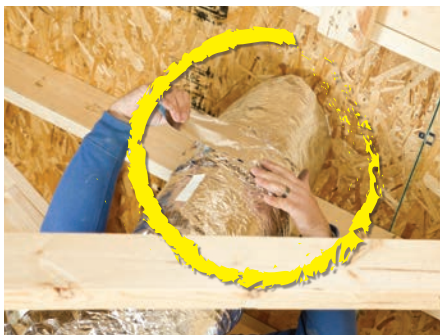
Insulate ducts that are located in unconditioned spaces.
